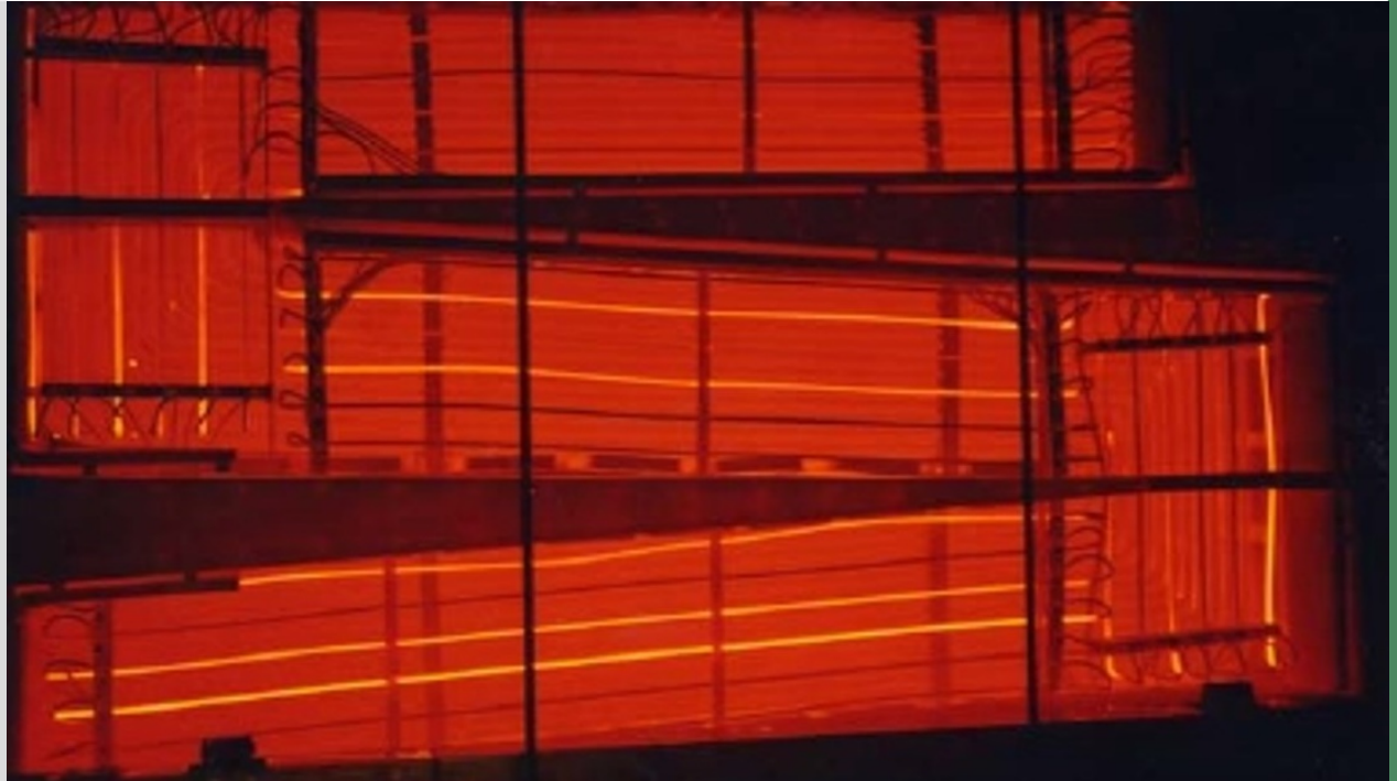
MSRE air-cooled radiator with its door open
