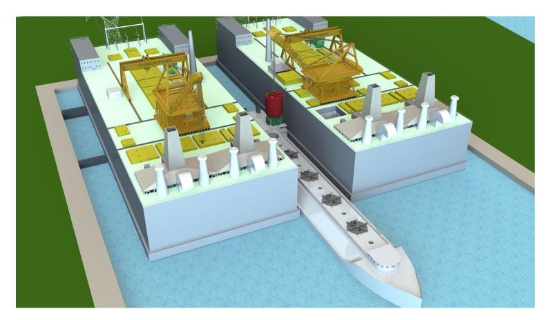
Plants are built complete in a shipyard, towed to a site in Indonesia, ballasted to the seabed, and then connected to the grid.
