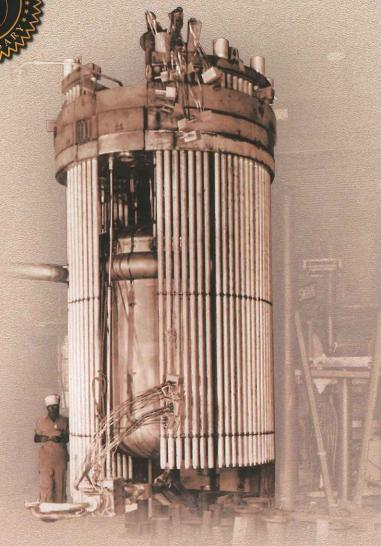
The MSRE was the result of a detailed research and development program in a number of engineering and scientific disciplines. A reactor mockup was constructed to demonstrate the feasibility of remote maintenance on highly radioactive systems. The MSRE was designated a nuclear historic landmark in 1994.
