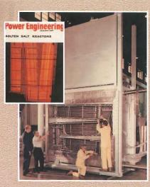
Heat was removed through this air-blast radiator (which glowed red when hot) and was dissipated through a metal stack to the atmosphere.
