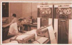
The main control panel displayed information that the reactor operator might need immediately, such as the temperature of the molten salt—if that temperature dropped below 840°F, the salt would begin to freeze. Computers and data handling equipment provided current information and analysis of variables within the reactor system and of potential abnormal conditions.
